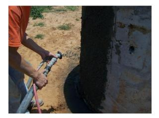
Sprayable geopolymer formulation for the rehabilitation of manholes and sewers.
