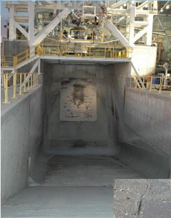
Test patch for Geopolymer Concrete
